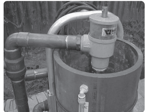
Figure 15: Cam Fittings for Flush Cart Hoses
