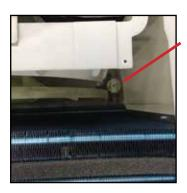
Thermostatically controlled drain valve allows defrost water to drain in heat mode.
