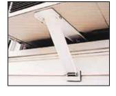
Both brackets install and remove with no structural disturbance.
