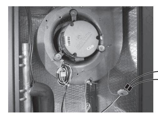
Note: Be sure to turn power off when removing and reinstalling harness to motor or damage will occur.
