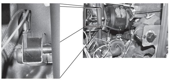
Verify 24V at reversing valve when calling for cooling
