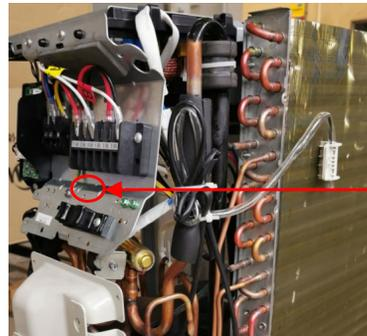
9) Remove the PCB board.
